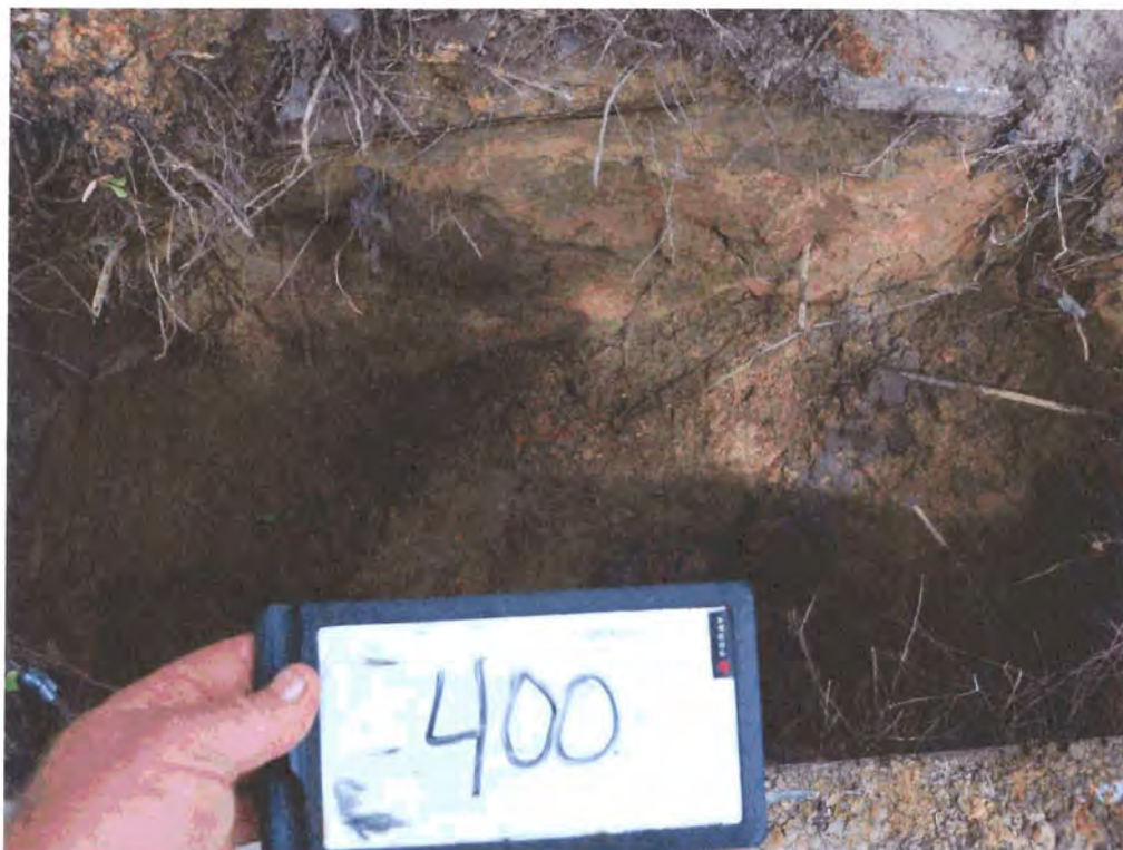
Picture 2: UST 400Elderberry excavation after tank removed.
